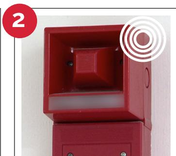
2 Using 'listen and learn' technology, the device learns the sound of the building's fire alarm.
